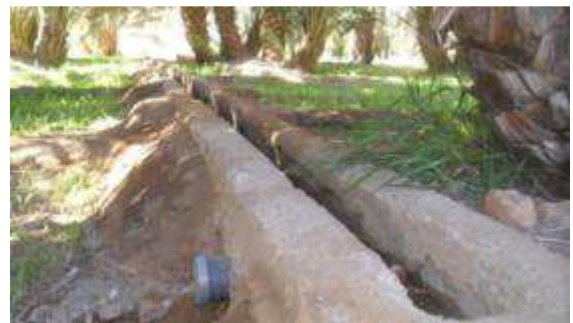
Figures 14: Uncovered Canals inside the Parcel
