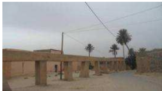
Figures 10: “ Saguia ” leading water to the basin
