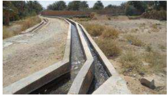
Figures 12: Uncovered canals
